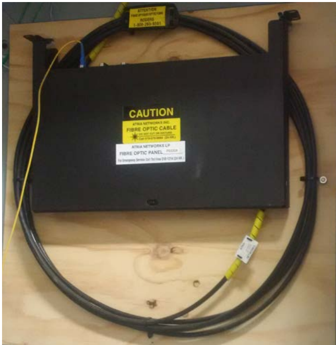
Above: Always leave several loops of spare cable in the control panel. Right: If a cable is being installed outdoors it will have a stronger jacket/armouring on it.
