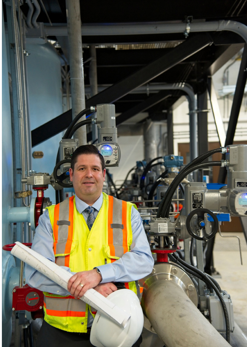
Graham Nasby, P.Eng. at one of the City of Guelph's newest water treatment plants (Guelph, Ontario, Canada). Photo by: Andrew Toms
