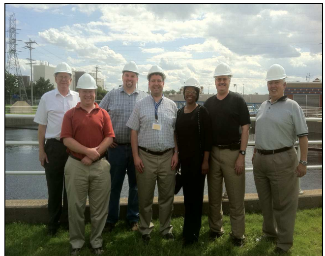
Photo of the tour group, taken in near the secondary clarifiers.
